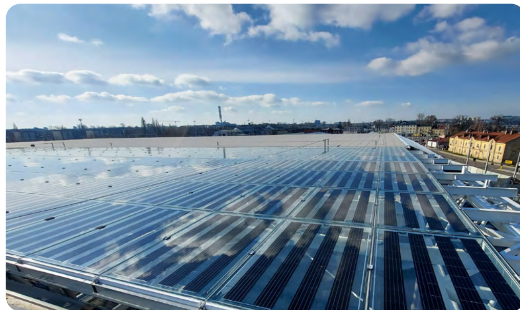
Lublin (PL) Bus station Roof with heated glass and LED lighting Output kW: 500
