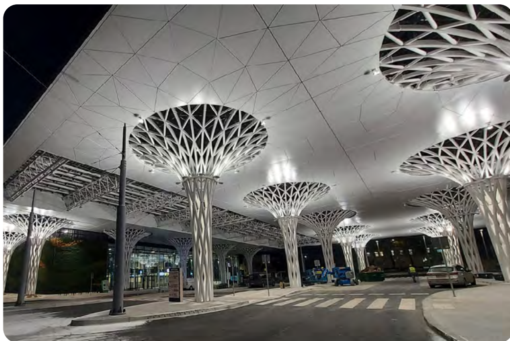
Lublin (PL) Bus station Roof with heated glass and LED lighting Output kW: 500
